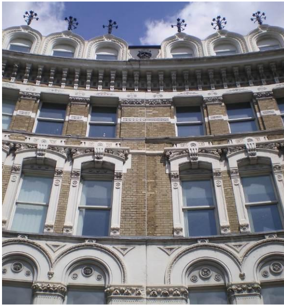
NE quadrant of Ludgate Circus
